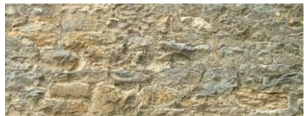
WALLING ('BUTTERED' STONE WALLING)
