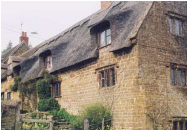
INAPPROPRIATE REED THATCH
