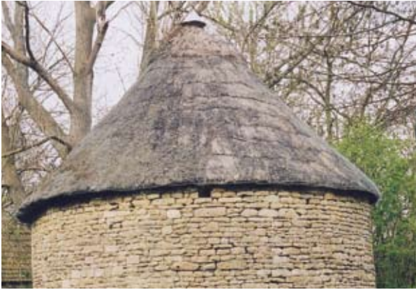
THATCH IN NEED OF MAINTENANCE
