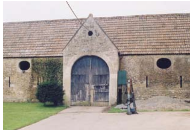
THATCH REPLACED BY PANTILES
