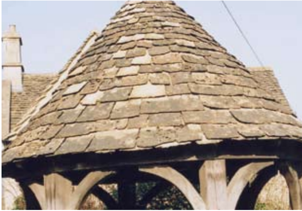
STONE SLATES IN NEED OF MAINTENANCE
