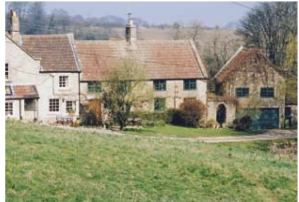
STONE SLATES REPLACED BY PANTILES
