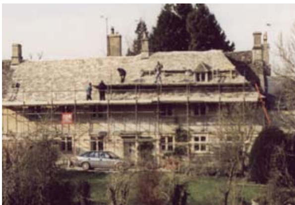
RE-ROOFING IN STONE SLATES
