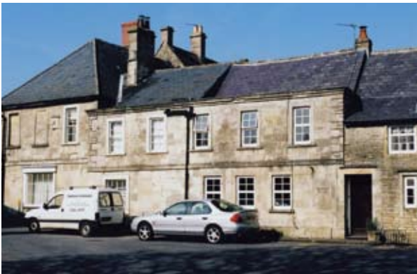
STONE SLATES REPLACED WITH WELSH SLATE
