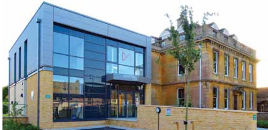
Mansion House with new main entrance building
