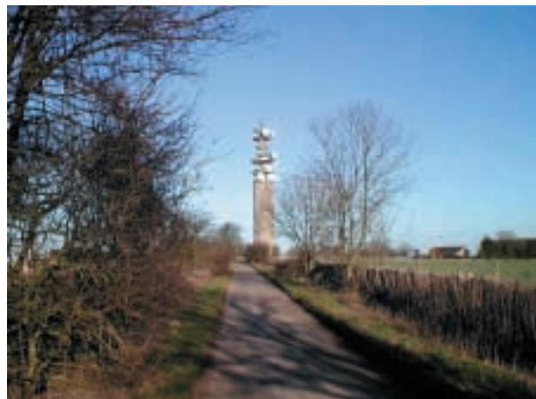
TELECOMMUNICATIONS MAST ON THE COTSWOLDS HIGH WOLD
