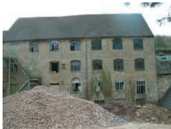
DERELICT MILL BUILDINGS IN THE VALLEY TO THE EAST OF NAILSWORTH
