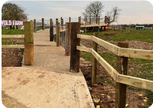
One of the new elevated walkways at the park
