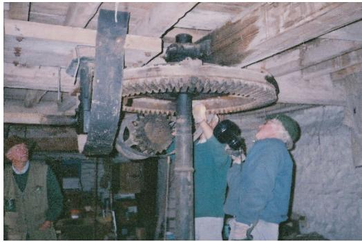
The next stage was to replace and knock home the wedges and hopefully the wheel would be true and would turn. Sadly, it would only turn 3" forward and back. They followed the transmission shaft to the first floor only to discover under lots of dirt and droppings, and behind screens and covers that a 9" square beam was resting on the horizontal crown wheel which supplied power to various pulley wheels. They thought this was the end of the line! With no
