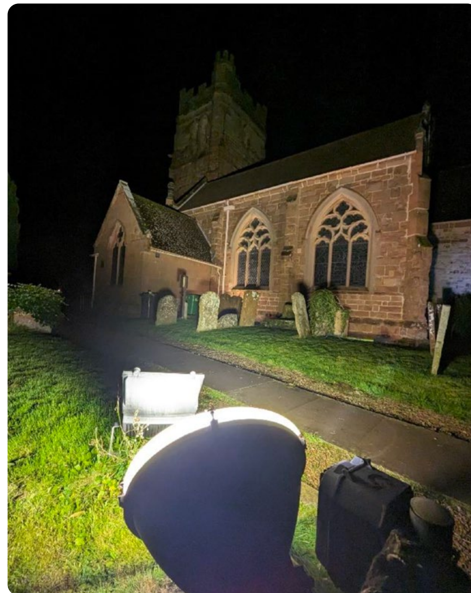
Figure 13 – How not to illuminate. Inappropriate luminaires used to illuminate a heritage asset (not in the CNL). Credit Dan Oakley
